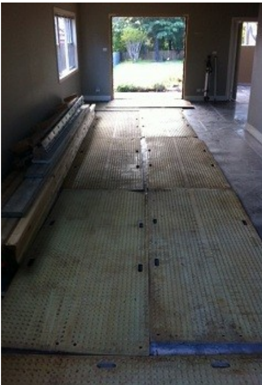
TrakMats used to prevent damage
