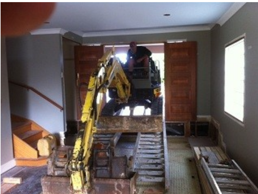
TrakMats used to prevent damage
